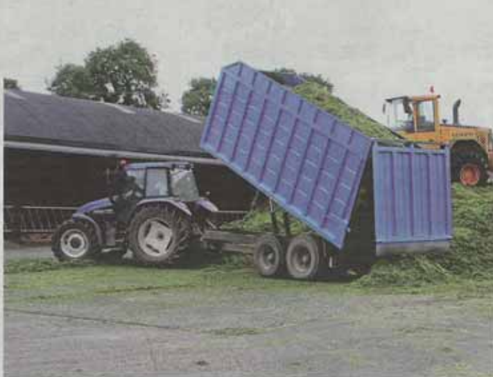
Silage effluent corrodes deeply into Portland cement concrete.
